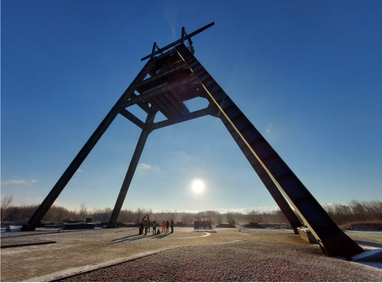
^ Barony A-Frame at Barony Colliery, Scotland. Photo courtesy of Dr Neil Burnside, University of Strathclyde
